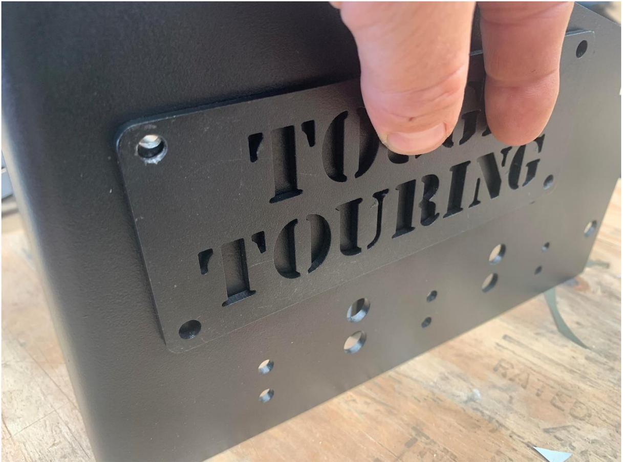
22. NOTE It is always better to measure twice and drill once! Take time and care to get the test fit straight and the rest of the installation will run smoothly. Get things square. Get them straight. Position all your brackets with test fit tec screws and open / close the tent to ensure you have the set up correct before you drill all the rivet holes.
